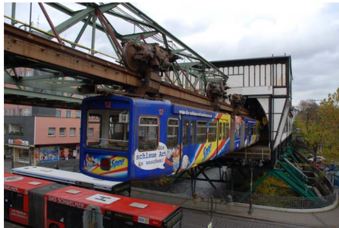
The suspended railway in Wuppertal.
